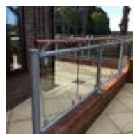
Glass Panel Balustrade
